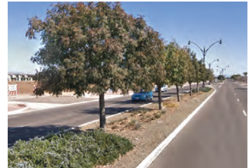
Designing for wider medians can accommodate plantings as well as turn lanes.
