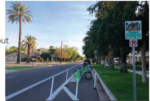
Flex zones allow for curb lanes to fill many uses, including, for instance, bike share docks.
