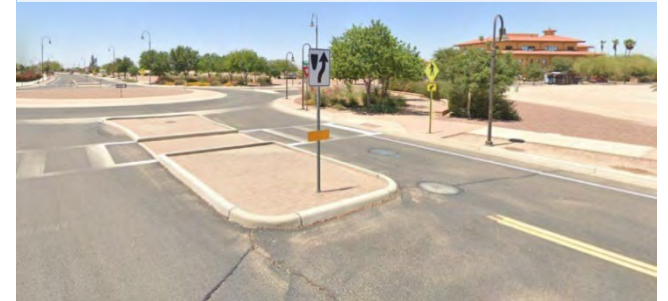
Pathway for people walking and biking from Greenberry Drive to Tangerine Farms Road in the Gladden Farms neighborhood
